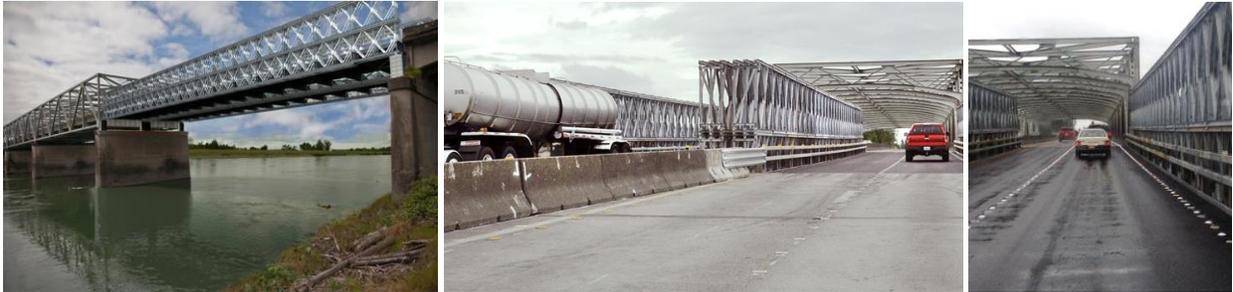
Figure 3 – WSDOT’s Skagit River Temporary Bridge (Acrow Bridge) – Triple-Double configuration
